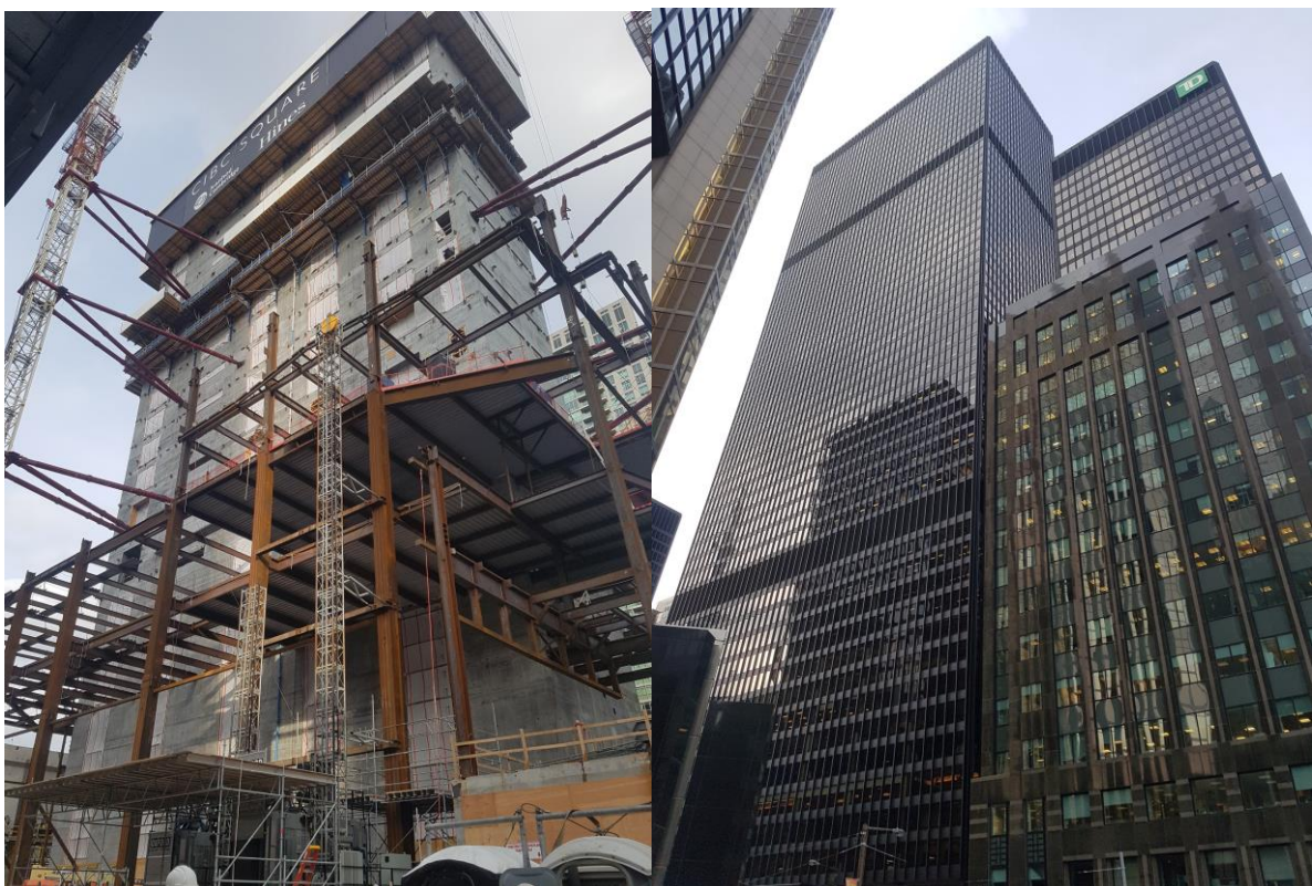
Figure 1.2 ( left) A photograph showing a new building under construction in downtown Toronto which is being erected in concrete and steel.
