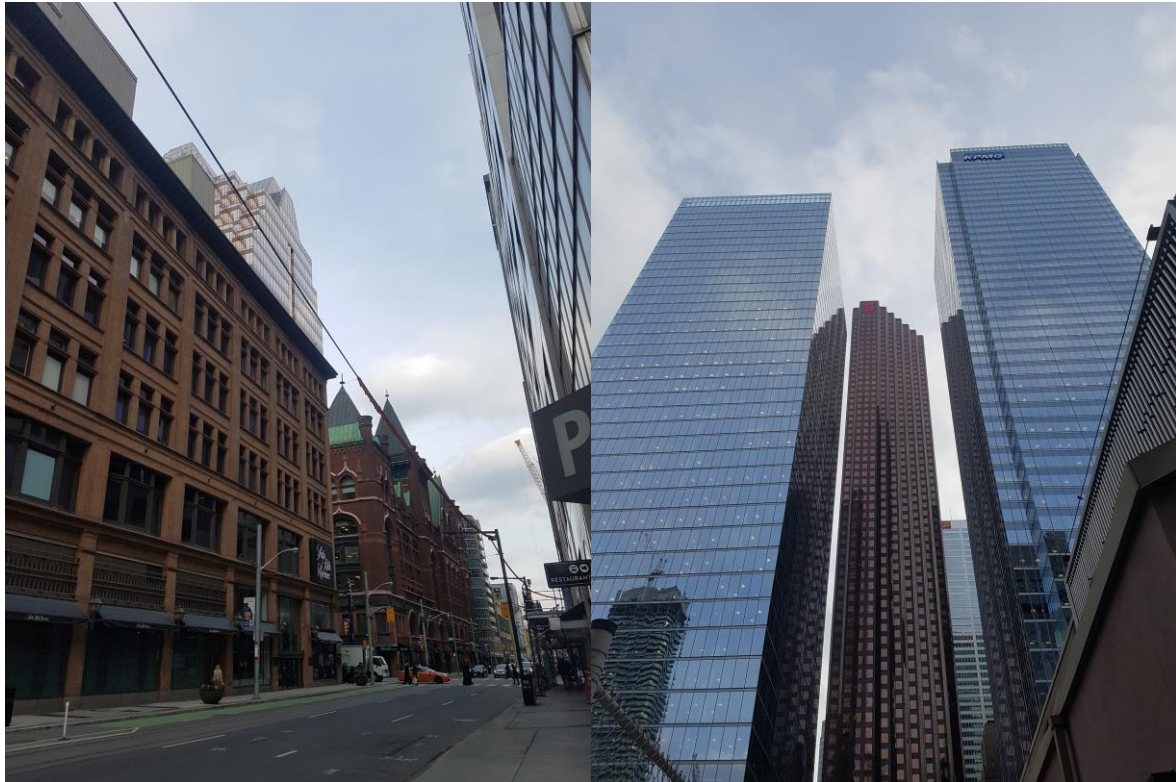
Figure 1.4 ( left) A photograph showing retail buildings in downtown Toronto built with red brick.
