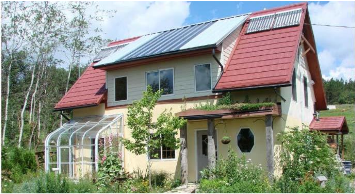
Figure 1.7: Photograph of 'Home Alive!' by 'Harvest Homes'. A 2 storey Straw bale and timber frame building located in rural Ontario, Canada.
