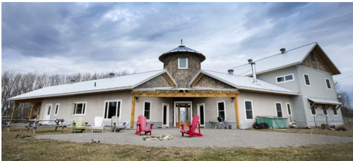
Figure 1.6 Photograph of 'Headwaters Farm House' built by 'Straworks'. A 1-2 storey Straw bale and timber frame building located in rural Ontario, Canada.
